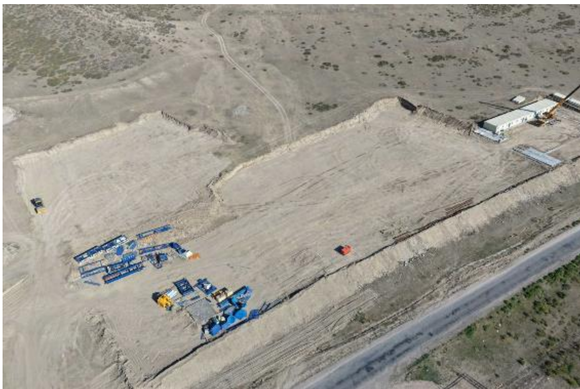
Figure 17: Removal of the topsoil on the territory designated for the development of the Production site of Section 2, km 202+220 RHS.
