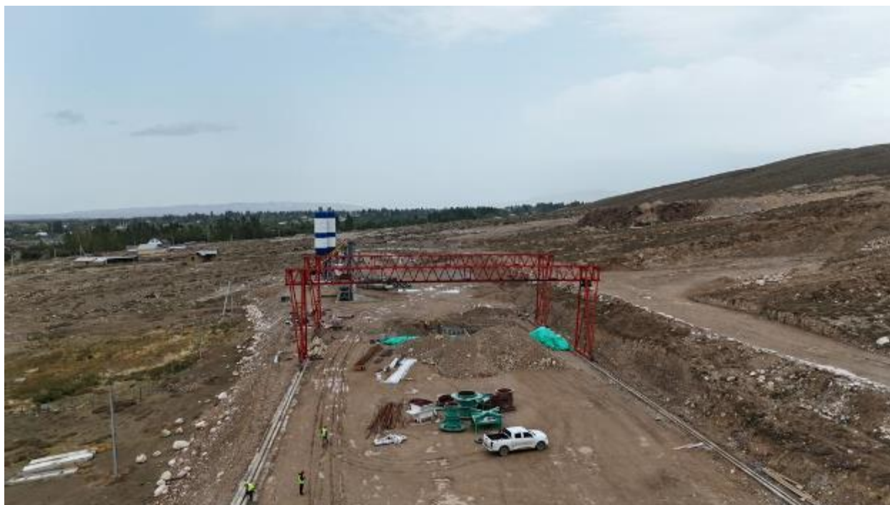
Figure 15: Removal of the topsoil on the territory designated for the development of the Production site of Section 1, km 167+360 RHS.
