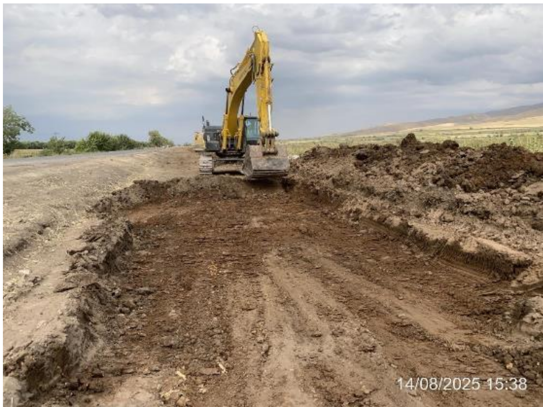
Figure 11: Removal of waterlogged material at km 188+800 (LHS).
