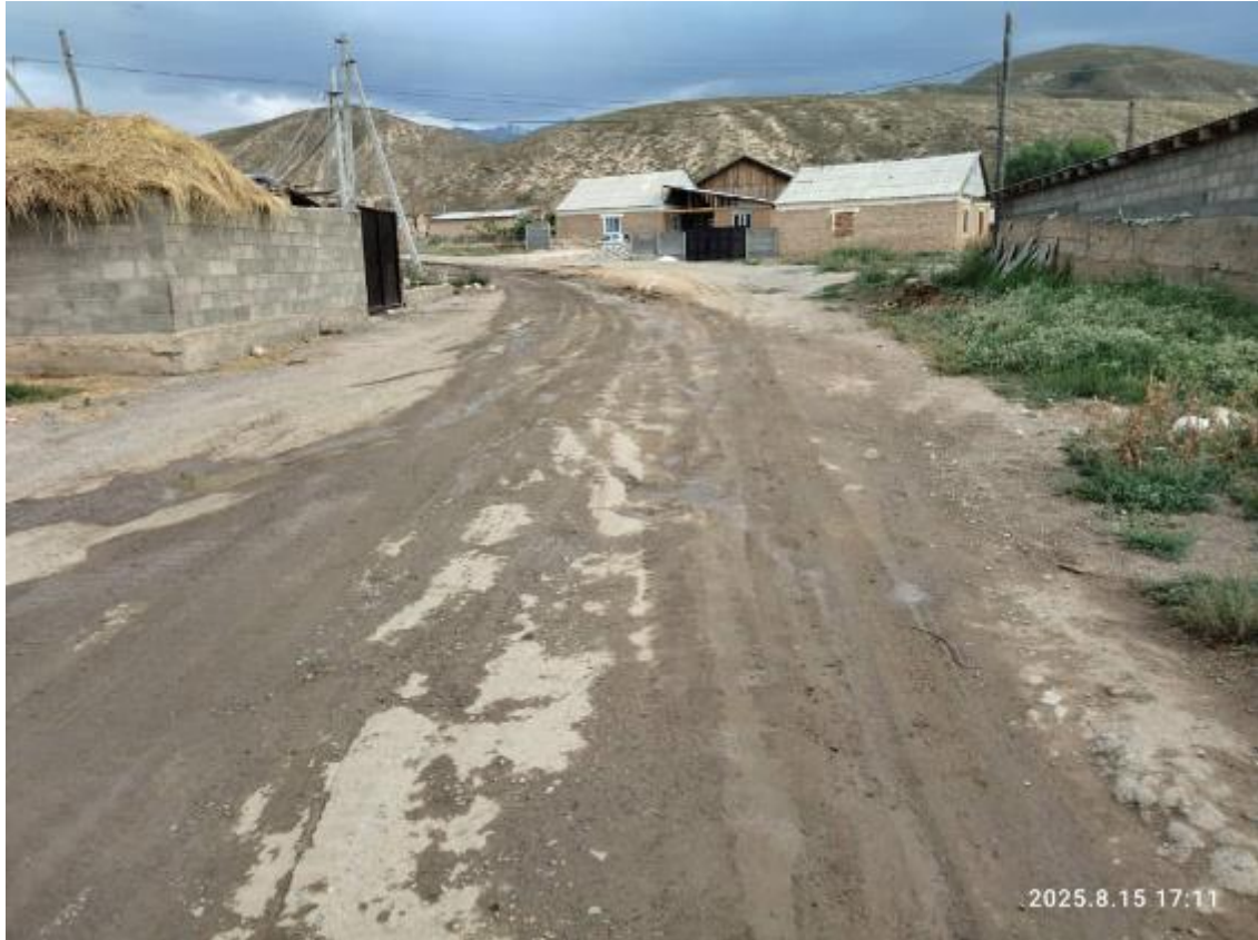
Figure 13: Km 152+580 dust suppression on access roads to the quarry is ensured.
