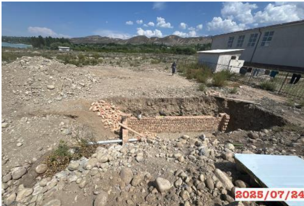
Figure 6: Camp in the village of Kichi-Jargylchak, km 150+610 (RHS), construction of a septic tank.
