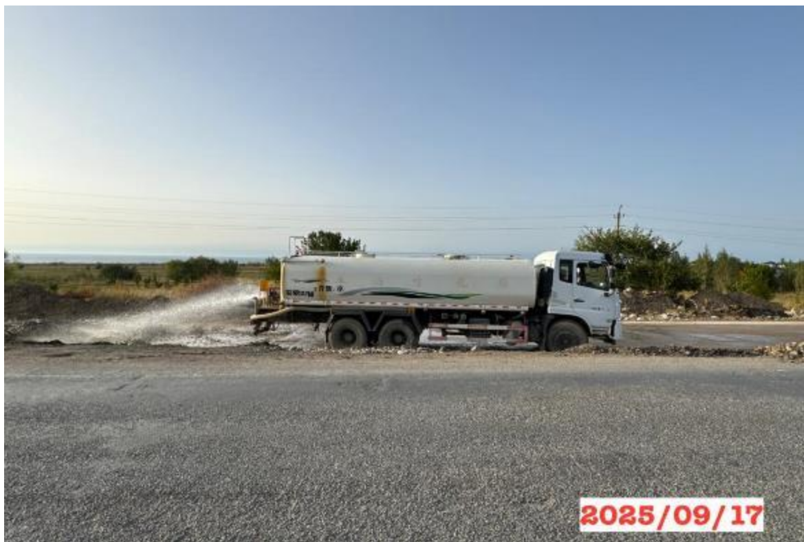
Figure 14: Dust suppression along the road is provided.
